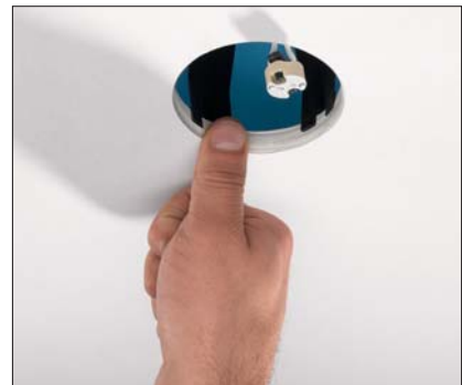
Push the retaining spikes into the plasterboard to prevent subsequent shifting.
